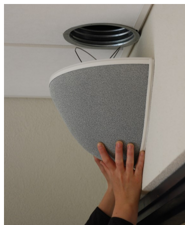
Image 3: Easy mounting with spring connection
